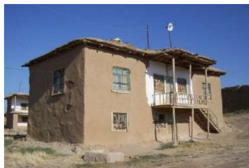
Figure 9: A brick house from Central Anatolia (Anulsin, n.d.)
