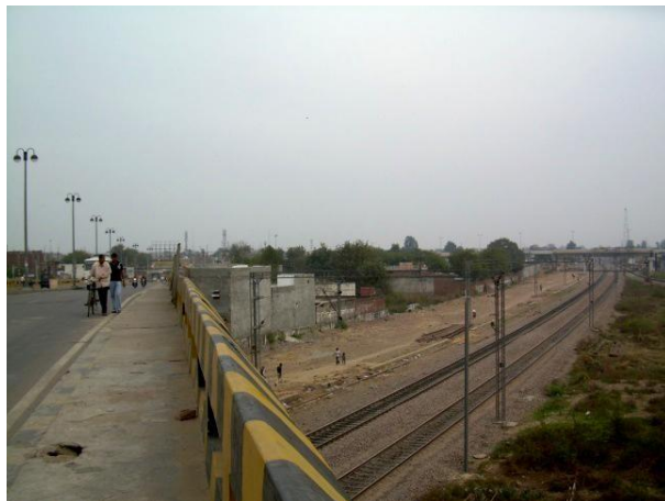
Figure 18: ROB over Rohtak Jind Railway lines
