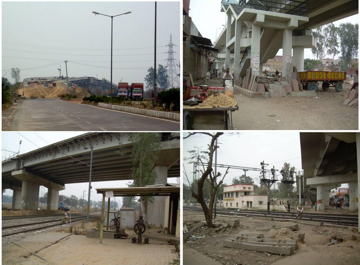
Figure 17: Construction of ROB in progress and completed ROB.
