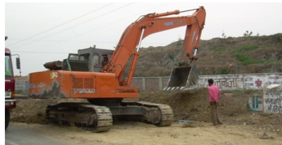
Figure 14: A view of Jind Road NH-71(2-Lanes)
