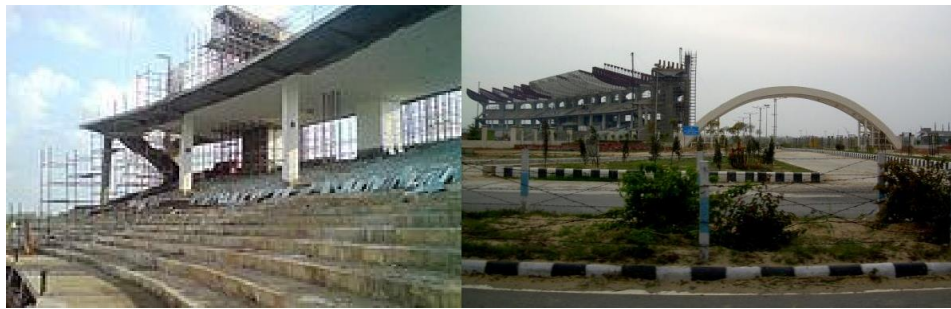
Figure 12: Construction of Athletic Stadium in Sport's complex.
