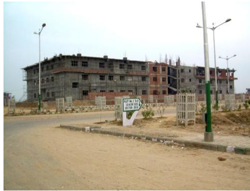
Figure 11: Phase- II - Under Construction.
