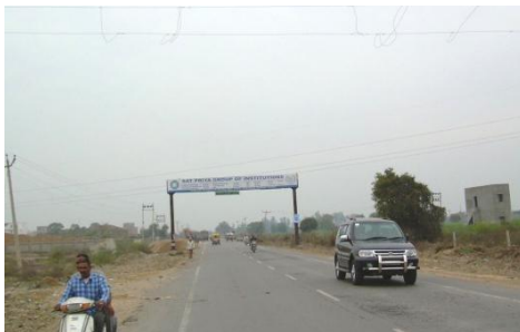
Figure 13: 4-Laning of NH-71 has started
