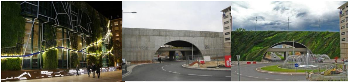
Figure 4.3 (left): Palace of Congresses Urbanarbolismo ( http://inhabitat.com 2015), Figure 4/4 (right): Bridge in France before and after ( http://twistedstifer.files.wordpress.com 2015, http://www.livingwallart.com 2015).
