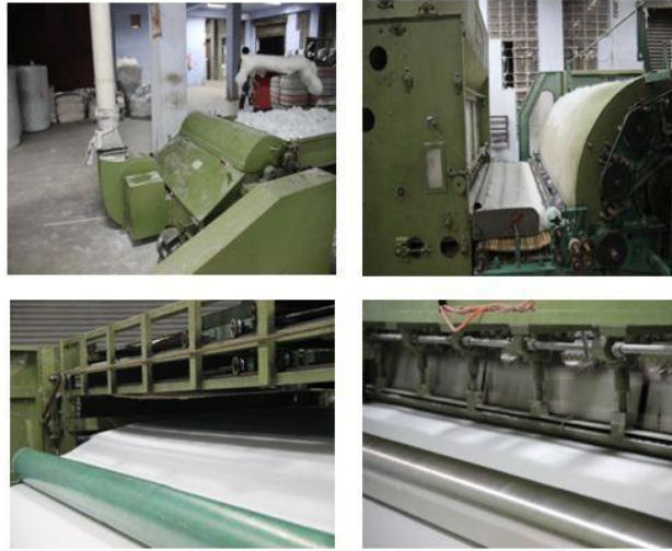
Figure 1: Actual Photo of various processes from actual site of ABC Company
