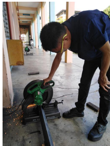
Figure 2: The Second Step was to cut the Metal Plate
